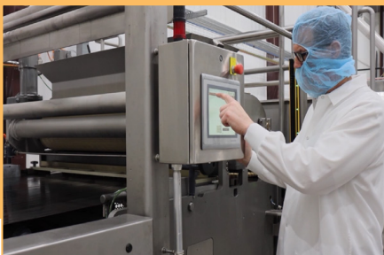
RBSCoConnect control panel
